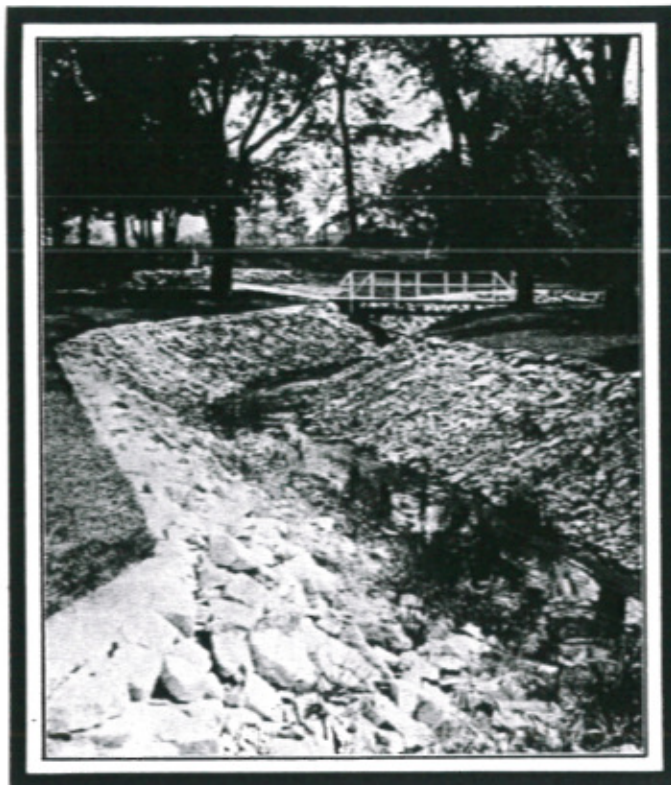
A completed drainage ditch.
